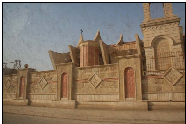
The church in central Qaraqosh. Photo: ACE
